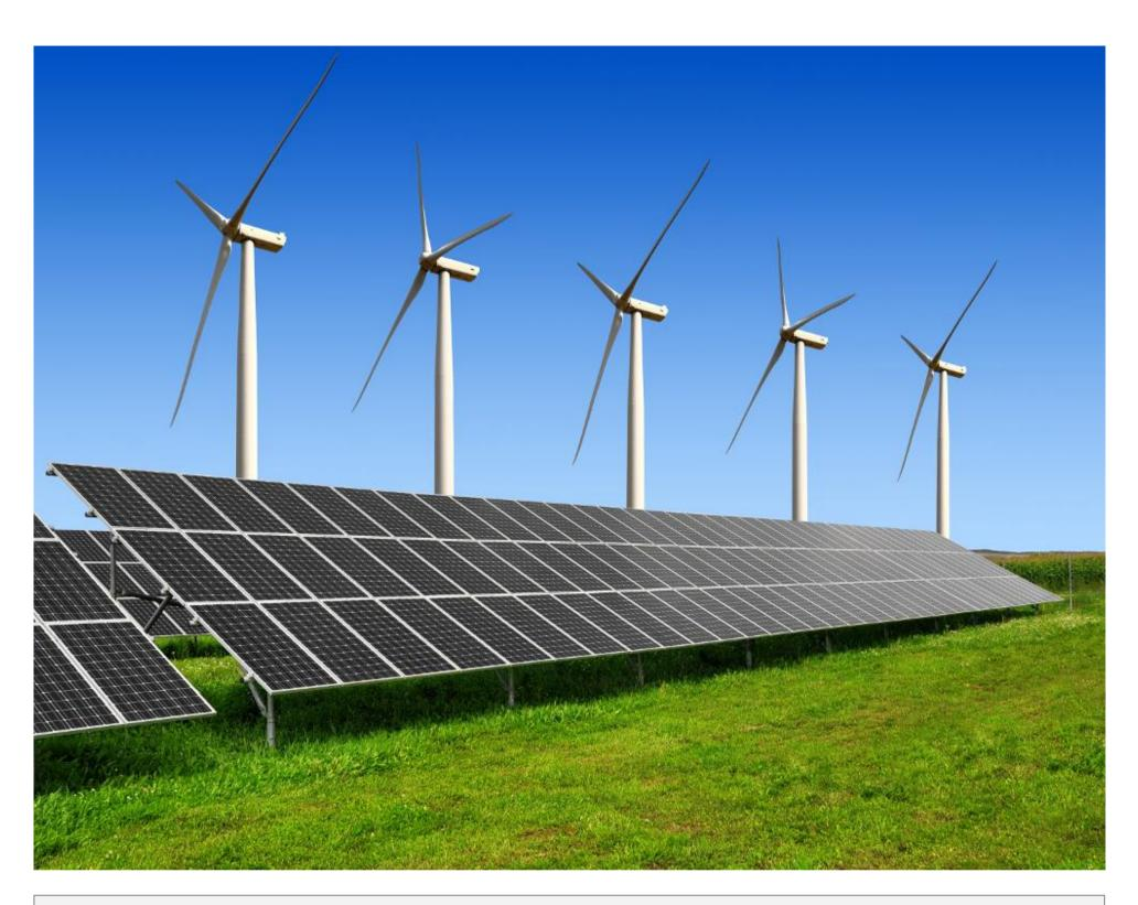
Solar-wind hybrids use solar panels and small wind turbine generators to generate electricity. They work in small capacities, typically in the range of 1 kW to 10 kW for the combined system of solar panel and the wind turbine.
